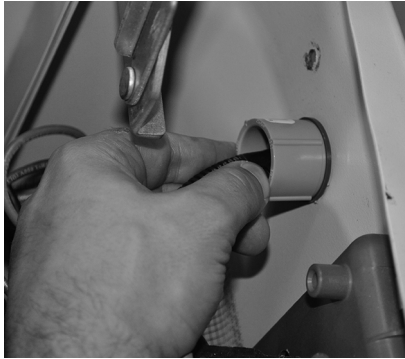
Figure 3.7 - Installing Fitting with Harness
