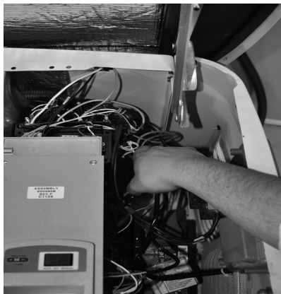
Figure 3.4 - Checking Wire Clearance
