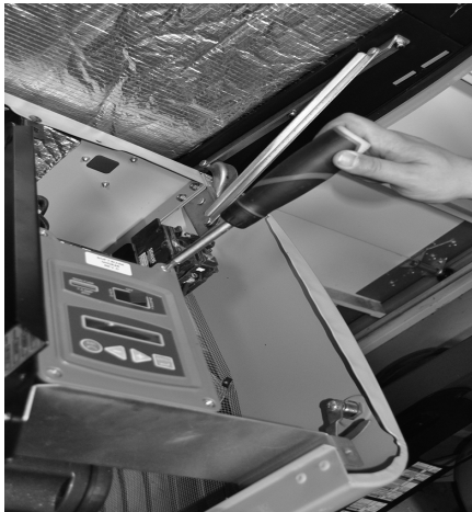
Figure 3.13 - Removing Controller Fasteners.
