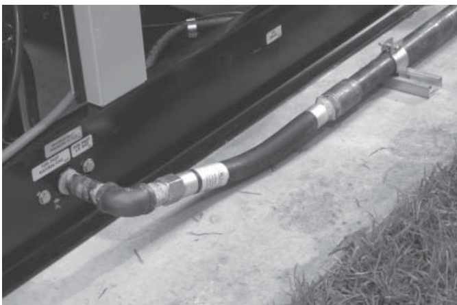
Figure 1.8 — Flexible Fuel Line
