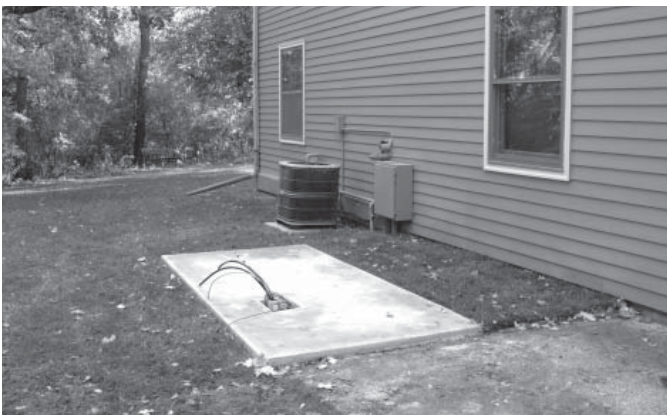
Figure 1.1 — Mounting Pad
