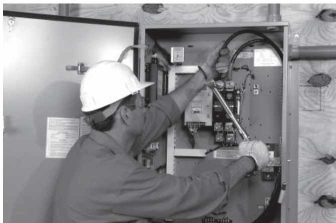
Figure 3.5 — Torque Lugs
