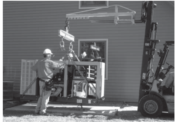
Figure 1.4 — Lifting the Generator
