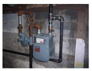
14) All of our natural gas-powered generator installs require a dedicated gas raceway from the gas meter to the generator. Tee tapping off an existing gas line to your furnace or hot water tank is not legal! Home Power Systems uses 1" minimum size gas piping to your generator. If you had a generator installed by another contractor, look at your install and see if it was done properly.
