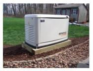
7) Generator install about 7' from home using pressure treated timber base. Notice that we use this install method when sitting in a bed of landscape mulch.
