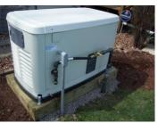
8) Home Power Systems underground install method for both natural gas and electrical raceways. Notice the gas valve is turned off for we are just finishing the installation. We use pre-manufactured gas sweeps for our installations, all direct buried utility approved.
