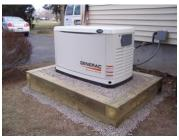
5) Another method sometime used for our generator installs. This customer wanted the generator to sit in the gravel, not directly on the timber base. This base also used two – 6"x6" timber bases for fear of high water that sometimes occur in her side yard.
