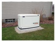
12) This install uses a pre-cast concrete pad called "The Gen-Pad". A new product that contours to the base shape of the generator creating a very neat and clean look for your Generac Generator.
