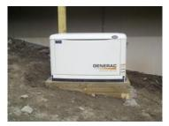
6) Professional generator installation on a very steep grade using 6"x6" pressure treated timber. Notice how it is strapped down to the base using prime and painted steel fasteners. Another time proven install method by Home Power Systems.
