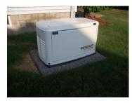
10) This is our standard install method using a 3" bed of pea gravel. We dig up the grass area, lay down landscape fabric and install the pea gravel. Very clean looking installation.
