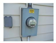
17) Every install requires us to install a "Warning Generator on Site" sticker on the electrical meter. This is to inform the fire department that there is a generator on site in case they have to cut your power.
