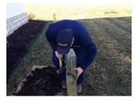
4) Here we are setting a 6"x6" pressure treated wood base. This method is used for pitched grades or when the generator is installed in a landscaped mulch area. Getting the generator off the ground, using the timber base, prevents rusting and allows you to use your power lawn trimmer and not damage the enclosure.
