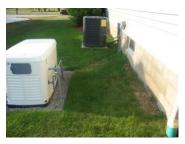
11) A side view of an underground generator installed 5' from structure. Electrical and gas raceways are straight and level at the generator and entering the house.
