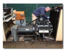
Our Commercial Power Systems division performs service and repair on larger generators as well up to 150kw. This picture shows an engine replacement under way on an older 100kw Generac generator. The fault was identified during a scheduled maintenance visit. Make sure your standby solution is maintained on a regular basis.
