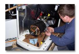
Commissioning and startup on your new Generac generator is the most important part of the installation. This engine is being replaced because the original installation contractor did not follow the proper break-in and start-up procedure. Home Power Systems follows section 3.1 "Break-In Procedure" of the installation Manual to assure longevity of your new power plant.
